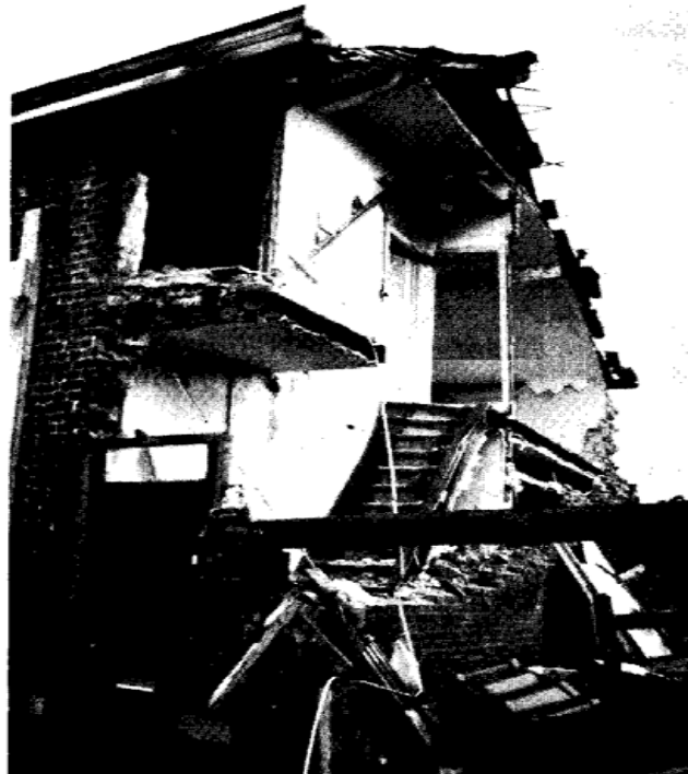
Figure 9 - Partially collapsed masonry building.
