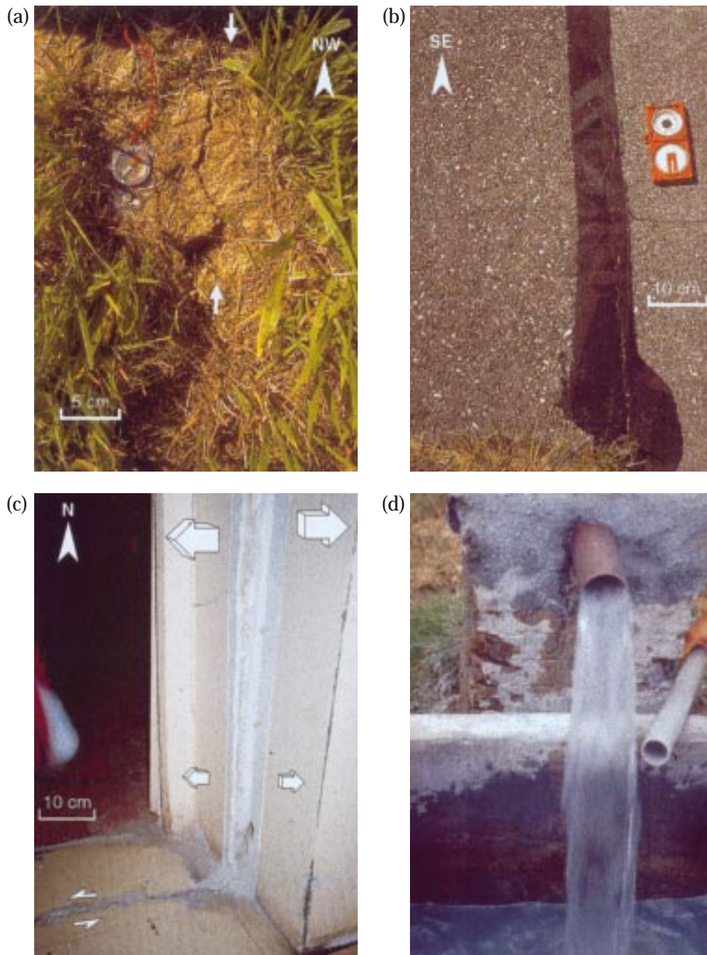
Figure 11. Ground cracks (a) a few metres west of and (b) on the runway of the Annecy–Meythet airport; see Fig. 7 (RC) for location. (c) Left-lateral strike-slip displacement at the Chaumontet warehouse; see Fig. 7 (CW) for location. (d) Output increase at Bromines spring, with old pipe and new pipe; see Fig. 7 (BS) for location.
