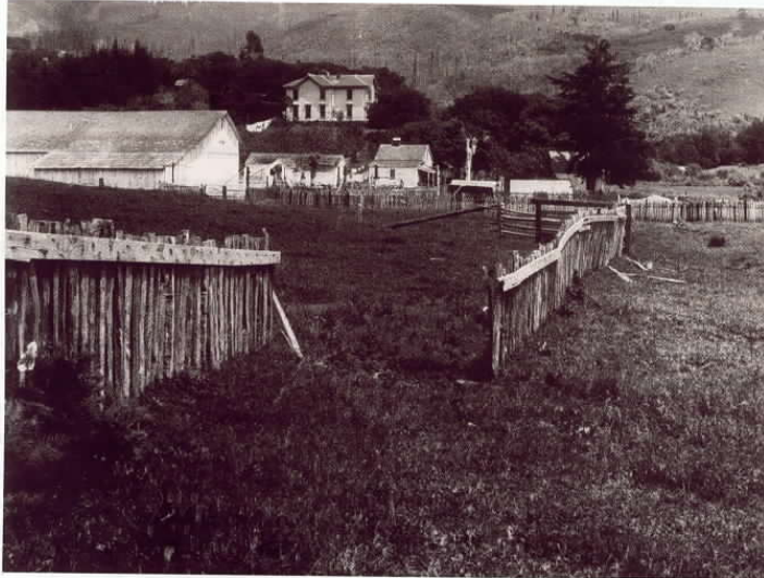
This fence running across the San Andreas fault in Marin County was offset 8.5 ft in the 1906 San Francisco earthquake as the land on the far side of the fault moved to the right.
