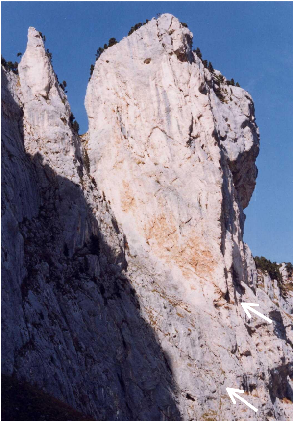
Fig. 2. Example of a potential rock slide in Grenoble area (height: 130 m; volume: 350 000 m 3 ); potential sliding planes are shown by the arrows. Smaller potential rock falls are visible on the upper right (overhangs).
